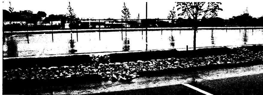
Bioswale within parking lot median
