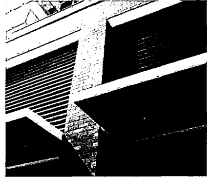
Soffit and Canopy
