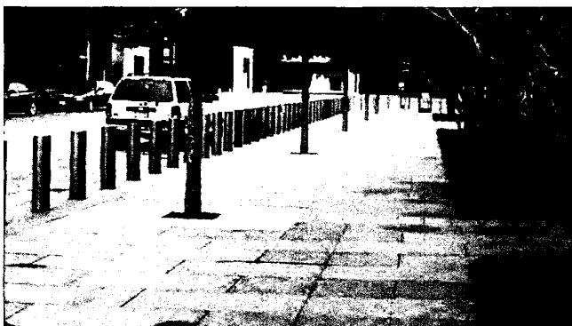
Stone pavers and tree grates along an urban streetscape
