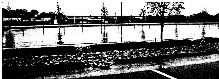
Bioswale within parking lot median
