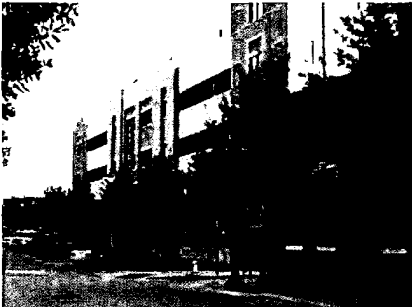
Trees lining parking structure and service drive
