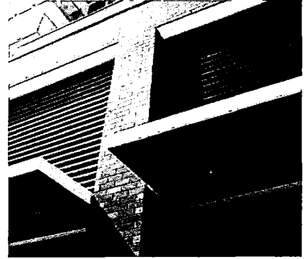
Soffit and Canopy
