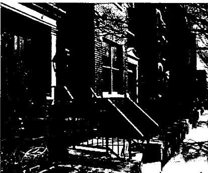
Landscape along front facades of townhouses
