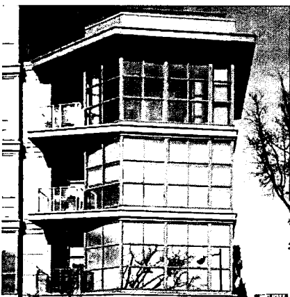
Section 5: Window Bays and Balconies
