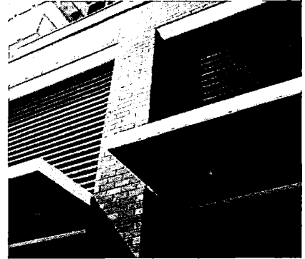
Soffit and Canopy
