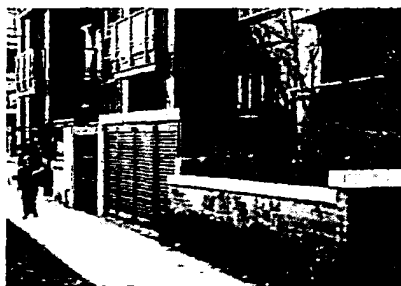
Example of appropriate screening with fencing
