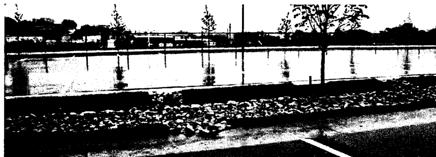
Bioswale within parking lot median
