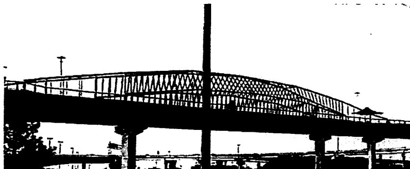
A trail bridge will cross Pacific Street to provide continuity between West Farm and South farm and improve public safety. The bridge will be a gateway element for the development.
