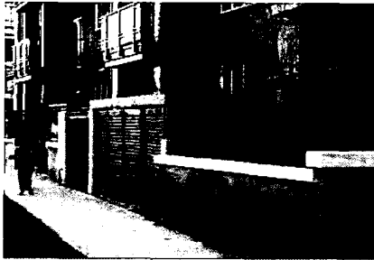
Example of appropriate screening with fencing
