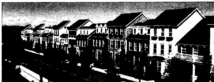
Example of building composition
