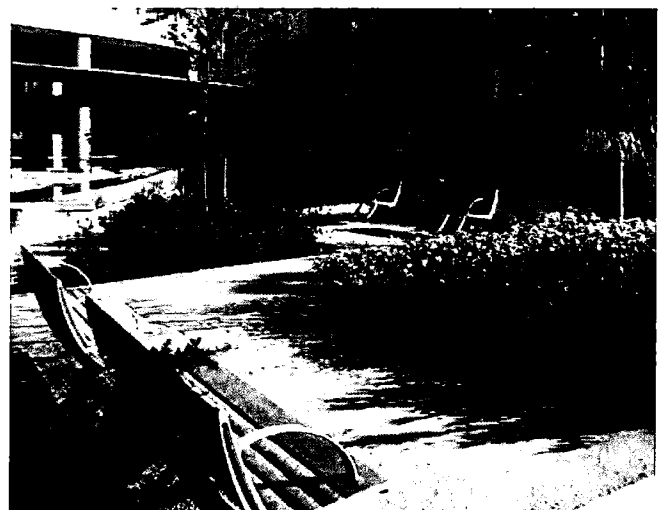
Crushed aggregate paving at small urban park
