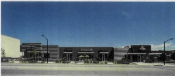
Push pull in the façade creating visual interest and individuality for retail tenants.
