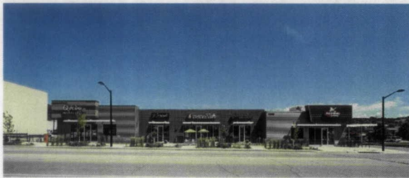
Push pull in the façade creating visual interest and individuality for retail tenants.
